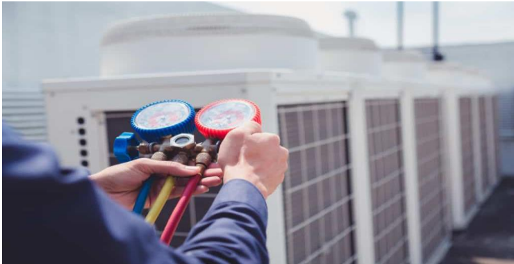
Technician checking HVAC systems
